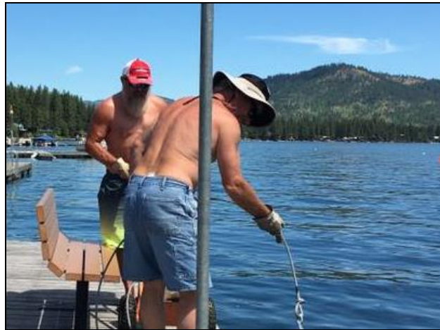
Rod F. & Rob D. installed 3 new anchors on Dock 3.
